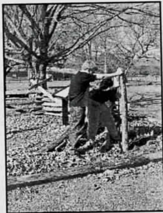
Jim and Nathan White work to install a post in the new (old) chestnut-rail fencing around the Civil War Trails sign behind the McDowell church
